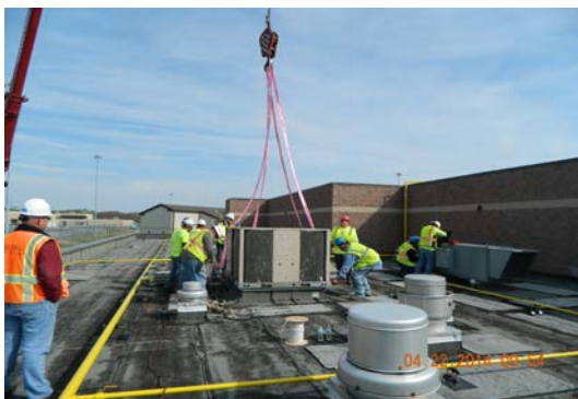
Figure 2-2 Vaughn Rooftop Unit Digging & Replacement
