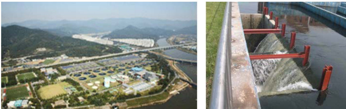
Figure 12. Shincheon sewage treatment plant and micro-hydro plant in Daegu (Source: Daegu Environmental Corporation)
